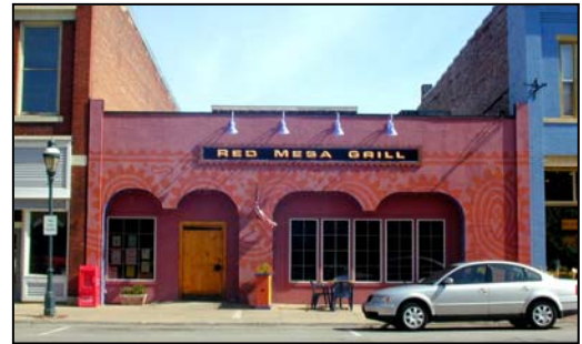
Though improvements to this building do assist in promoting the business's image, they are not in keeping with proper historic preservation building rehabilitation standards and support a false architectural style in downtown Boyne City.
